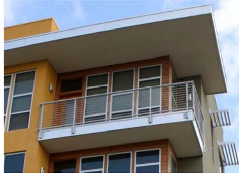
A Balcony is a private personal open space serving as access to light and air above the ground level. Metal or slab balconies may project out from the building face, be semi-recessed, or completely recessed. Balconies must be surrounded by guard rails or a building face. A balcony typically has French or sliding glass doors leading out onto it and can be entered from living room or bedroom.
