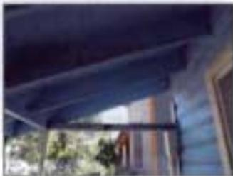
**Front porch:** A 2/12 pitch partial width shed roof projects from a 2"x10" ledger board attached to the exterior siding of the primary façade.
