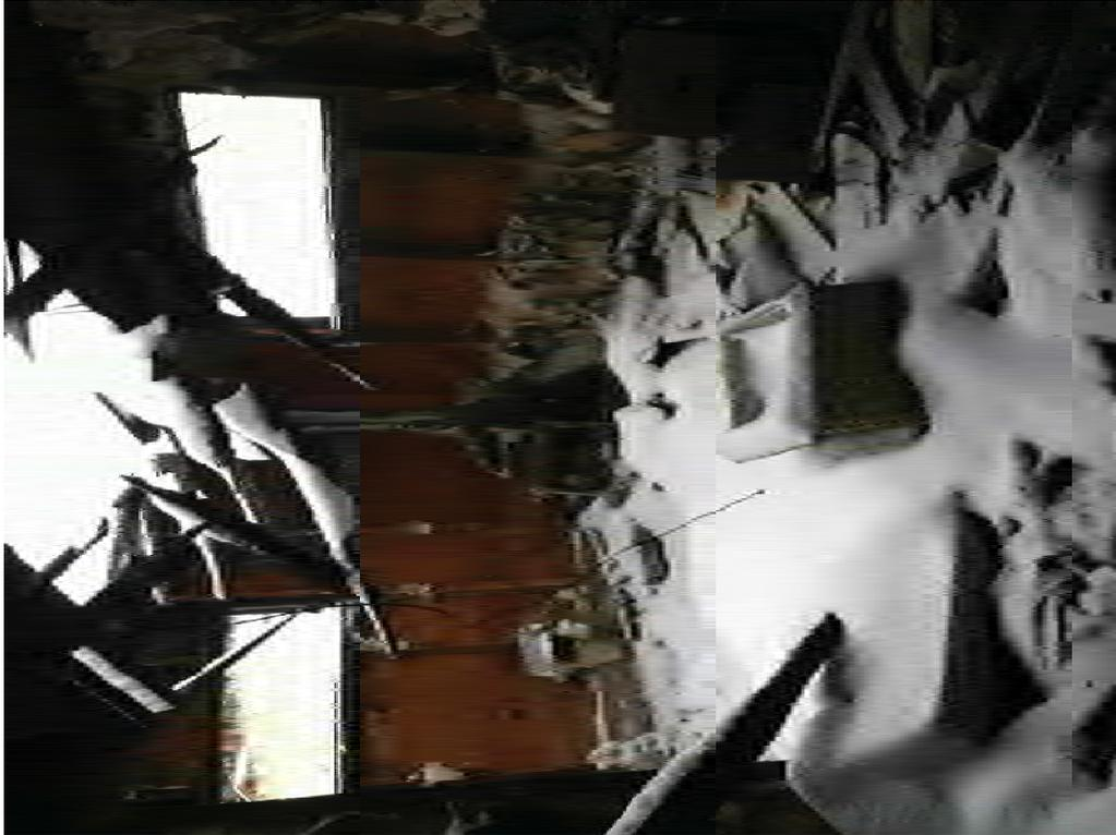
*Fire-damaged rear addition. Note the horizontal lumber atop vertical studs.*
