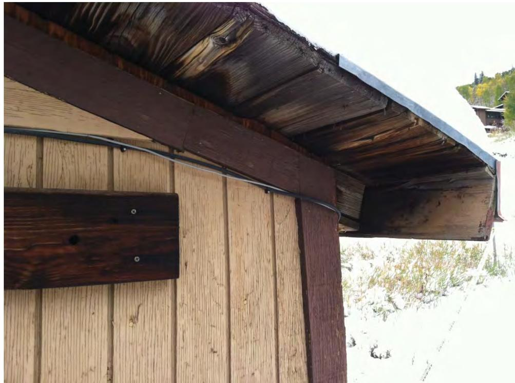
*Exposed roof eave, showing old growth timber*
