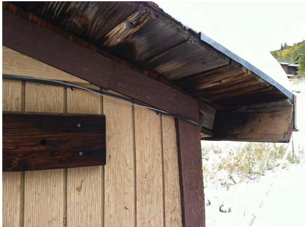
*Exposed roof eave, showing old growth timber*
