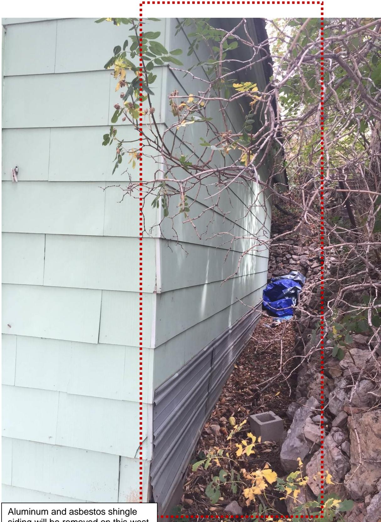
Aluminum and asbestos shingle siding will be removed on this west wall to determine condition of original wood siding beneath.
