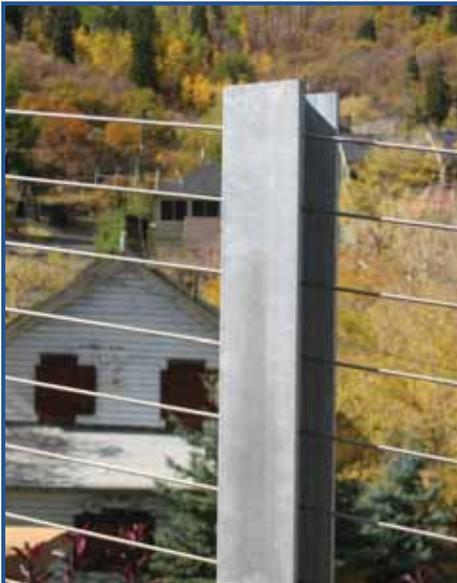
8 feet tall safety fences will be located at the top of protected retaining structures. They will be constructed of galvanized I-beam posts that are spaced 10 feet apart. The fences will be strung with 3/16 stainless wire with 3-1/2 inch spacing. Located uphill from these fences, where appropriate and as directed by Park City Mountain Resort, will be 12 feet tall, treated, painted black, 4x4 wood posts set in 2 feet deep concrete, located 30 feet apart with 3/4 inch galvanized eye-
