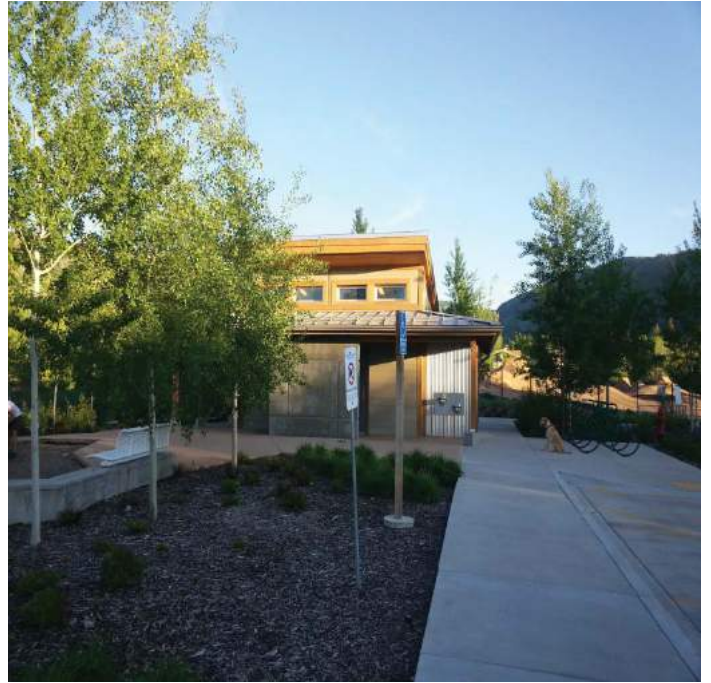
View facing south
