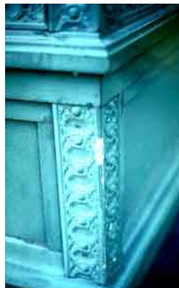
**Substitute materials need to be located with care to avoid damage. The fiberglass column base has chipped, whereas the historic cast iron would have remained sound. Photo: NPS files.**
