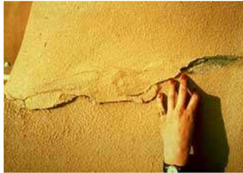
**A waterproof coating is an inappropriate substitute material to apply to adobe as it seals in moisture and may result in spalling. Photo: NPS files.**
