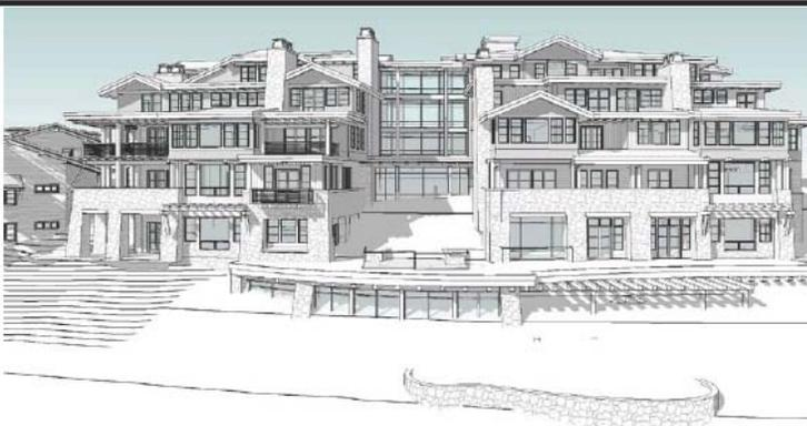
The current design minimizes the amount of exposed excavation and allows less disturbance to natural grade
