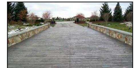
'Wood' Stamped Concrete for Bridge Element
