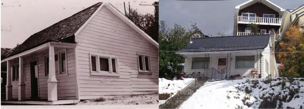
**37 Hillside Street:** *Modifications to historic porch, exterior materials, window-door configuration, construction of new chimney.*
