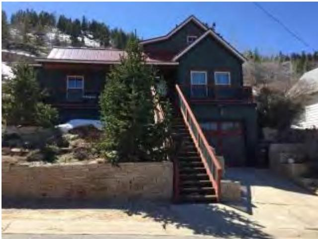
**347 Woodside Avenue.** Addition is not visually separated from historic structure when viewed from the Public Right-of-Way. Also, the addition of a window well on the Front Façade is inappropriate.
