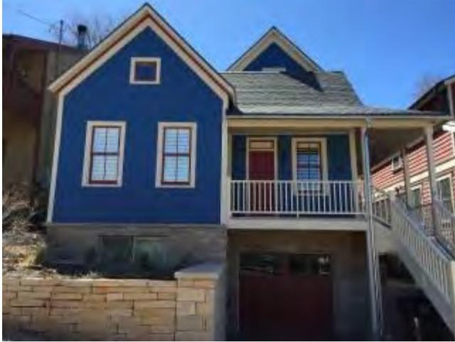
**951 Woodside Avenue.** Addition is not visually separated from historic structure when viewed from the Public Right-of-Way. Also, the addition of a window well on the Front Façade is inappropriate.
