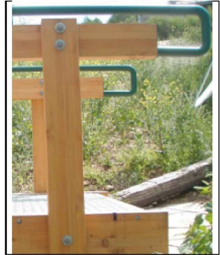
**IBC 1009.8 Stairway Landings** "There shall be a floor or landing at the top and bottom of each stairway. The width of landings shall not be less than the width of stairways they serve."
