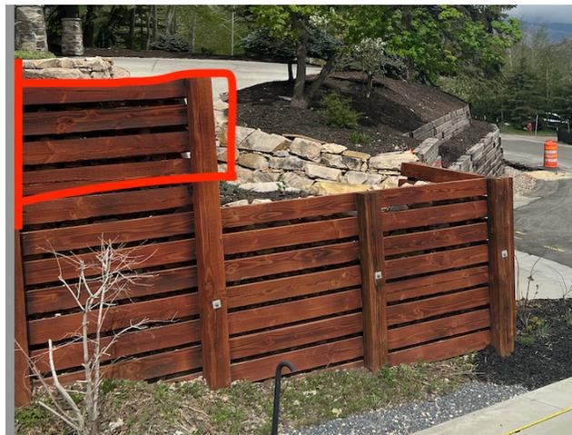
Picture 2: Retaining wall section higher than 4ft.
