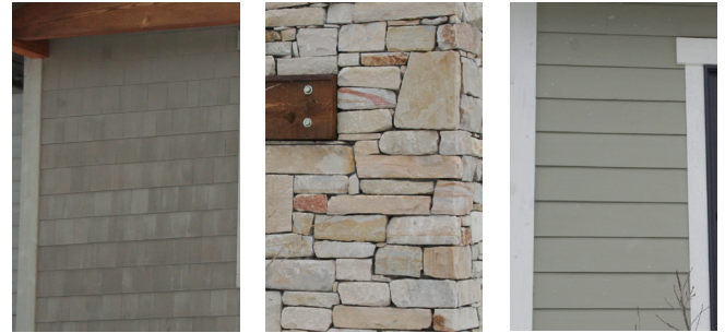
Varied wall materials provide interest and distinction to wall planes
