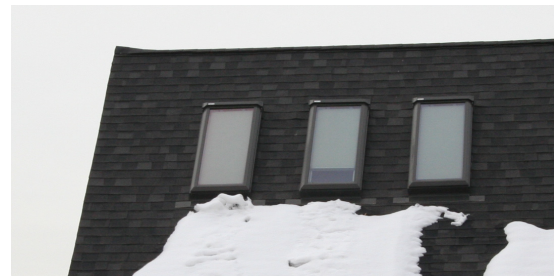
Skylights are flat to roof and do not extend to eavelines or roof peaks
