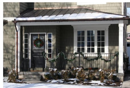
Porches are elevated 18” above finished grade
