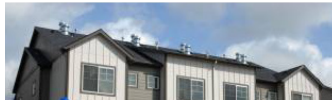
Mechanical vents reflect architectural style
