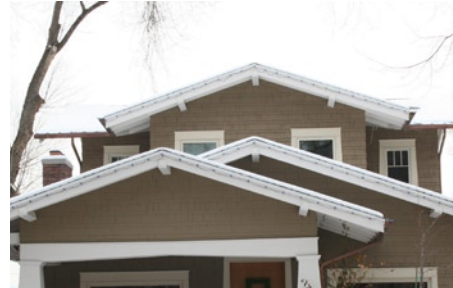
Appropriate roof overhangs
