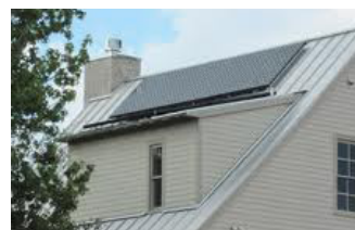
Solar panels located to minimize visual impact
