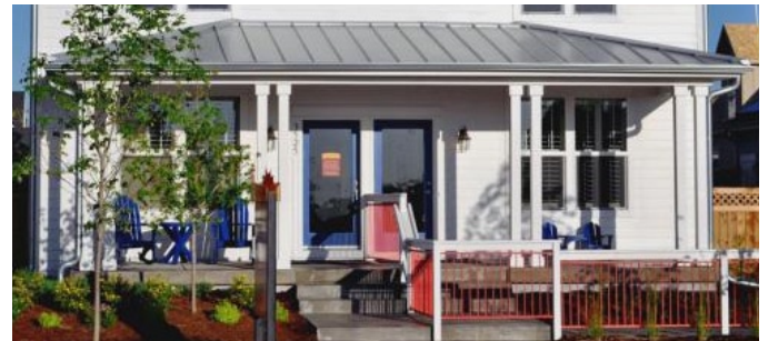
Properly detailed porch elements
