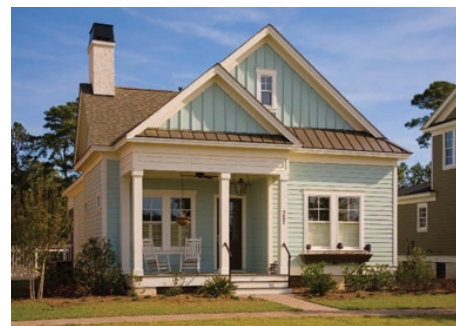
Porch roof forms are consistent with home
