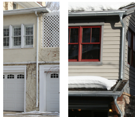
Gutters match trim or are appropriate for the architectural style
