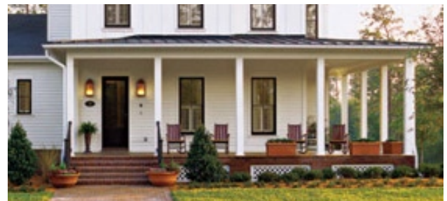
Porch raised a minimum of 18” above finished grade
