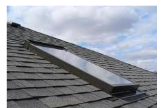
Skylight placed flush to roof
