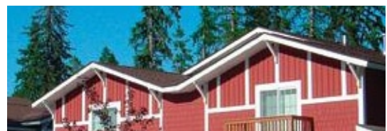
Roof is broken up to relate to human scale
