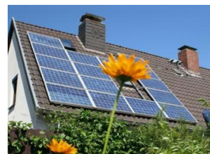
Solar panels visual impacts are minimized
