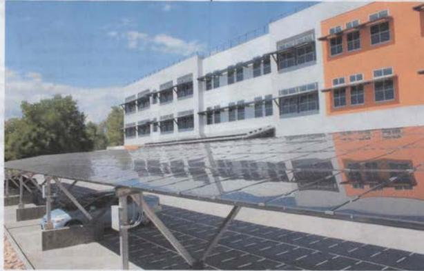
In addition to a remarkable collection of microbreweries, Fort Collins has deliberately set out to be an incubator for deployment of renewable energy and reduced-energy use buildings. This building has a net-zero energy use, helped by the use of solar collectors over parking spaces.
