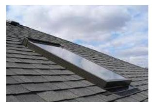
*Skylight placed flush to roof*
