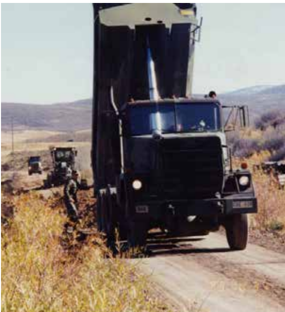
Construction of the Rail Trail
