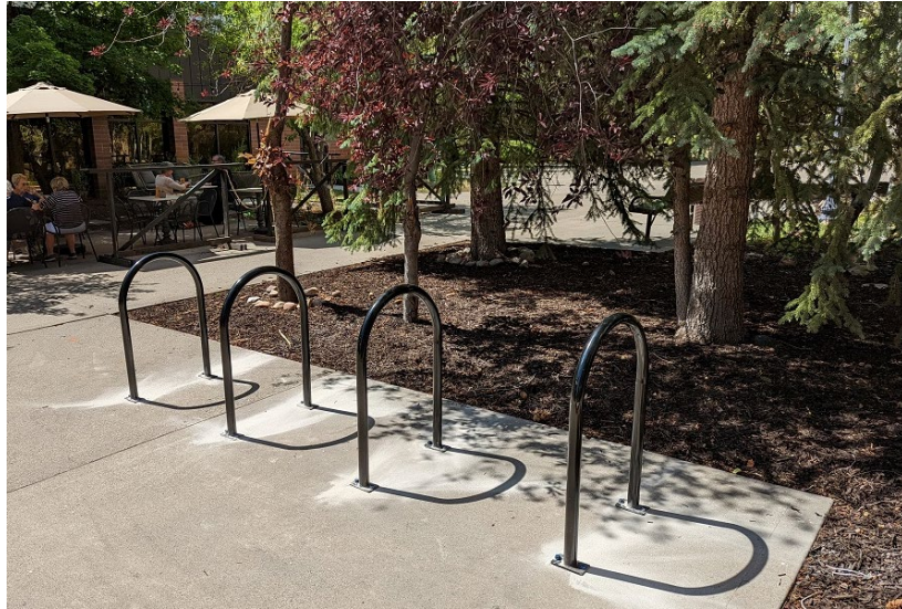
Saltbox Bike Rack Install
