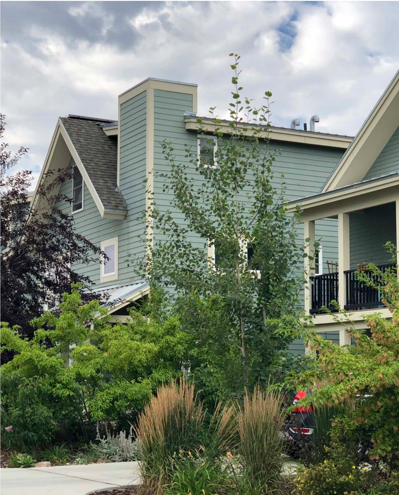
Snow Creek Cottages Affordable Housing
